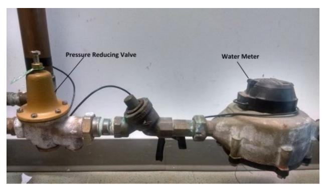
Because of the Town's topography, we have higher pressure in our mainlines than a lot of systems. The PRV helps reduce that pressure before the water enters your home. Most household plumbing is not suitable for higher-pressure water systems, requiring a PRV.
