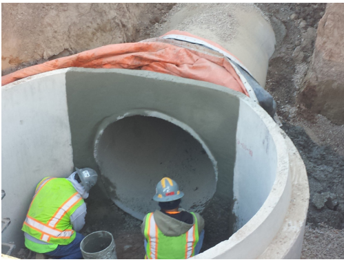
Garfield Storm Sewer and Modeling, Wellington, CO
