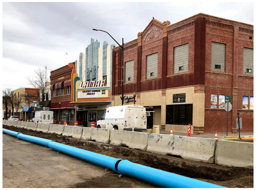
Main Street Waterline Replacement, Lamar, CO
